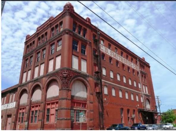
The now vacant C.D. Smith Drug Company building is Edward's Family warehouse.
